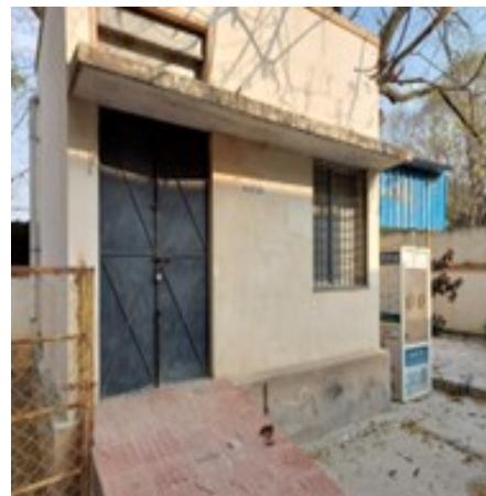
Locked Mortuary Room at CHC Kengeri
