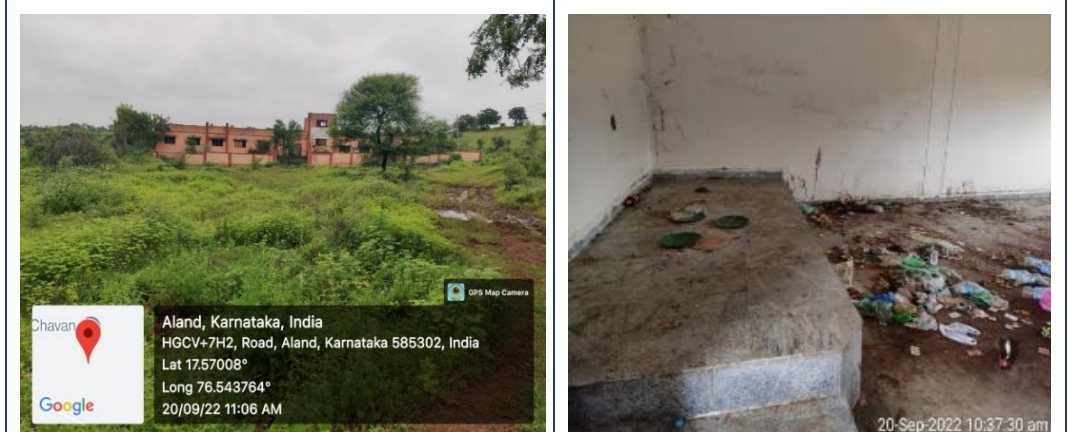
Government First Grade College at Aland constructed under Special Development Plan was found abandoned giving room for anti-social activities
