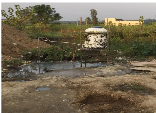
Unhygienic Drinking Water facilities at work site
