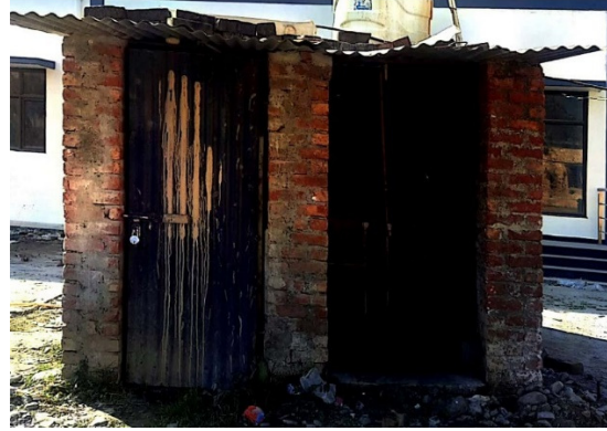
Defunct Latrine and urinals at worksite
