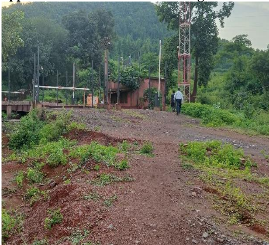
Photograph No. 1: Non availability of approach road at Lahanda Checkgate
