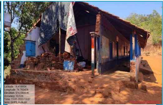
Condition of building in GHPS, Hulkurthi, Sirsi, Uttara Kannada
