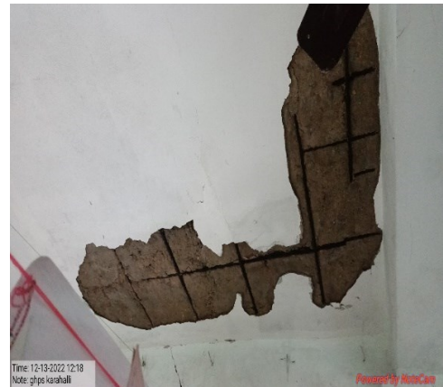
Condition of roof in GHPS Karahalli
