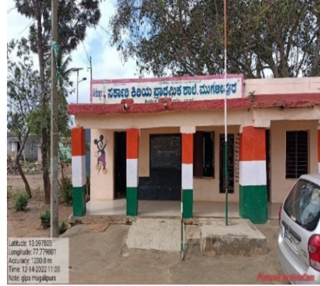
Poor condition of ramp in GLPS, Mugalipura
