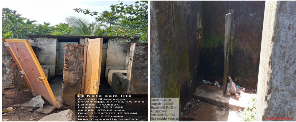
Toilets without door in Shivamogga
