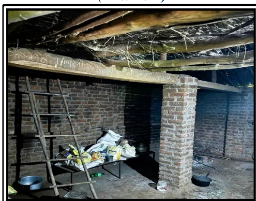
Picture 3.3: AWC with a dilapidated thatch roof (made of plant material) AWC: Parvadi 3, Godahra, Godhara (11-09-2024)
