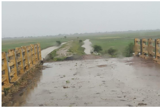
Image 3: One side of the bridge (Kumhra side) remained unconnected (as of 30.09.2021), with the 3 km length of road, having been constructed on other side of the HLB (Laxmipur side)
