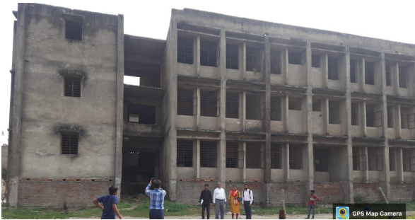
Image 1: Incomplete building of SDH, Manjhol, Begusarai
