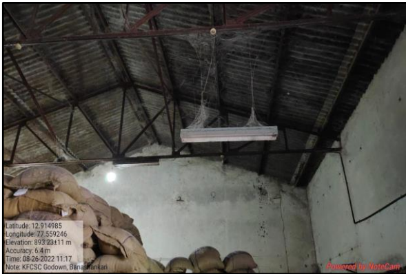
Old dusty ceiling which is made of asbestos sheets - KFCSC Banashankari, Bengaluru South IRA
