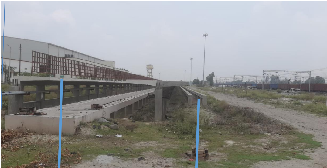
First washing Pit
