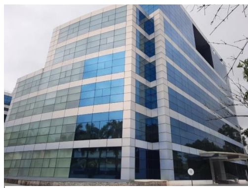
Figure 3.7: QuEST Global building at Technopark Campus, Thiruvananthapuram
