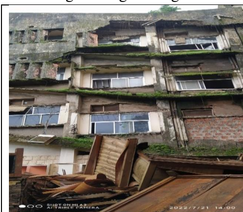
Photo No 3.1: East side of Academic Block
