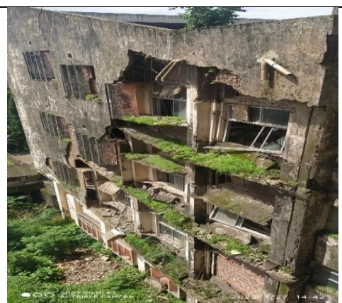
Photo No.3.2: West side of Academic Block
