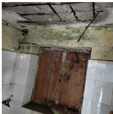
Image 5.2: Damaged roof of the toilet of PHC, Noorsarai (23.05.2022)
