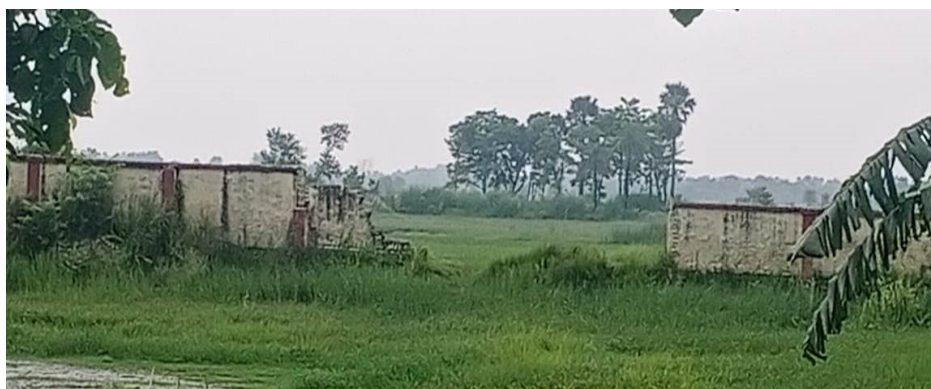
Picture No. 4.1: JNV Vaishali- Demolished compound wall
