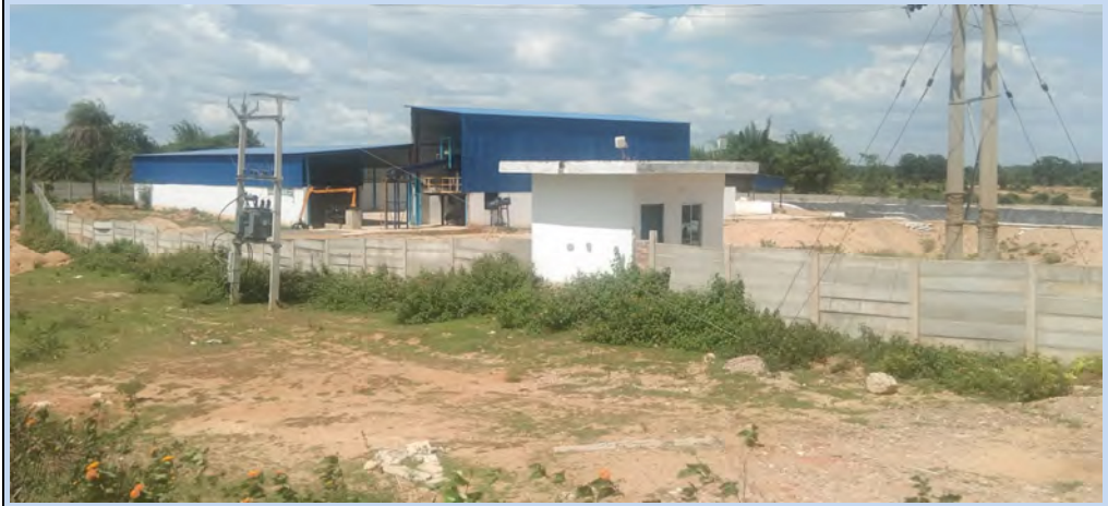
Exhibit 7.2 : Construction (including landfill site), at the Jhumritelaiya & Koderma cluster MC, without obtaining EC (photograph taken on 23 November 2022)
