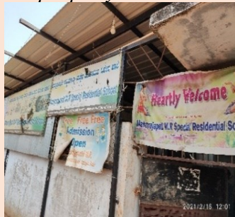
Residential School Building
