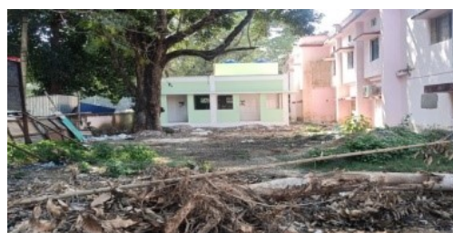
Picture-21: Toilet without approach road at SDH, Karanjia
