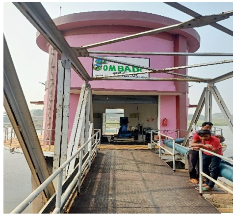
Picture-7: RCC structure intake well
