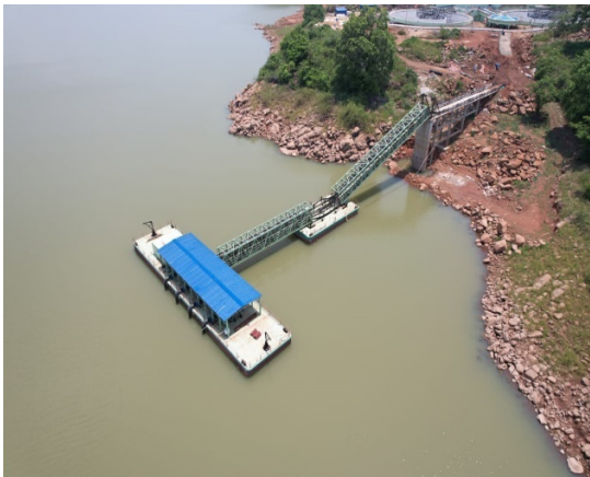
Picture-6: Floating jetty type intake well
