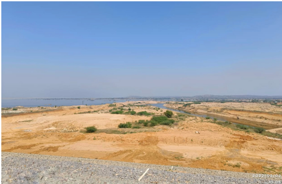
Figure 4.4 - Submerged Feeder Channel inside SKMS Reservoir
