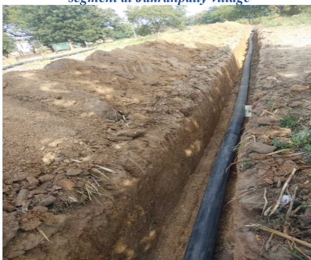
Figure 6.1 - Laying of HDPE pipeline in Metpally segment at Jakranpally village
