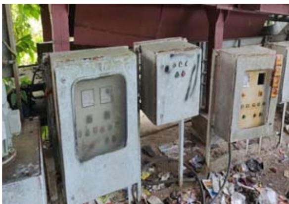
**Exhibit 6.9: Damaged panel board of compost plant**
