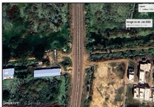
Picture 2.15: Western Bye pass road crossing through railway line
