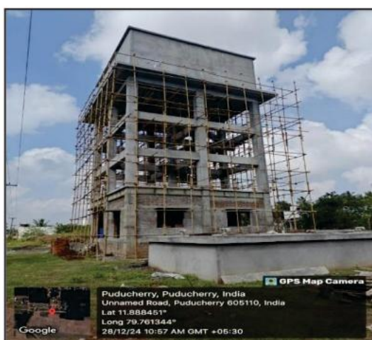
Picture 2.11: Slow progress of work in Thirukanji
