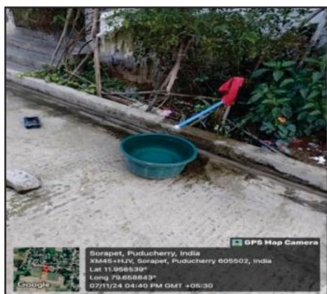
Picture 2.8: Provision of FHTC outside of house
