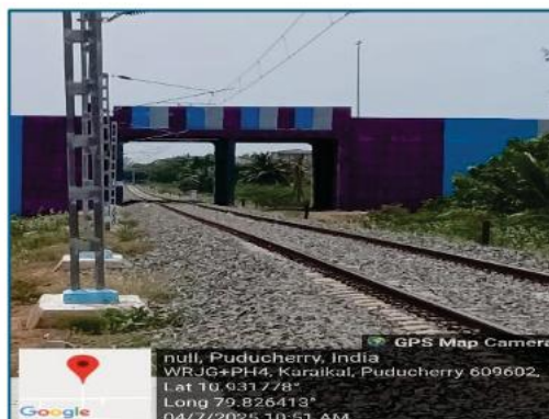
Picture 2.16: After the completion of RoB
