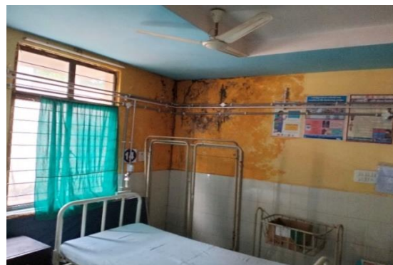
Figure 5.7: Seepage in ward at AH Seethampeta (June 2022)
