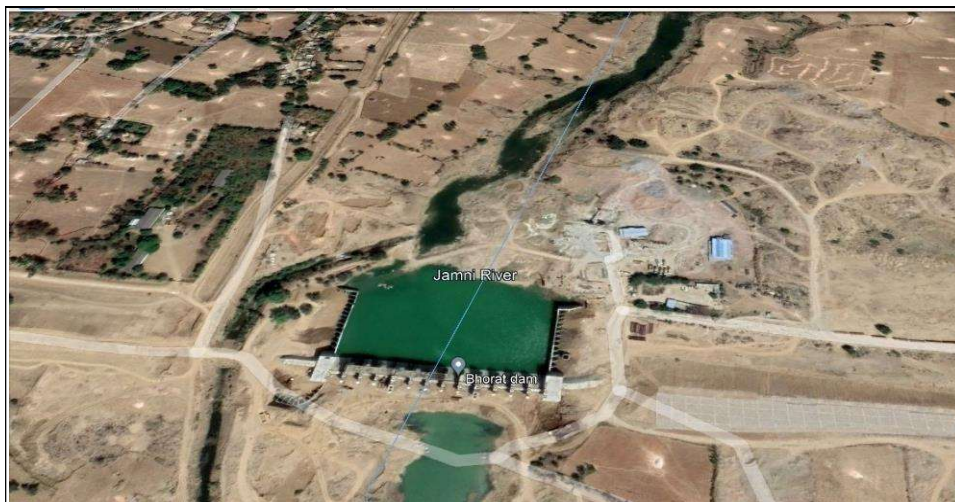
Image 3.1: Construction of Bhaunrat dam in District Lalitpur (dated 06 April 2021)
