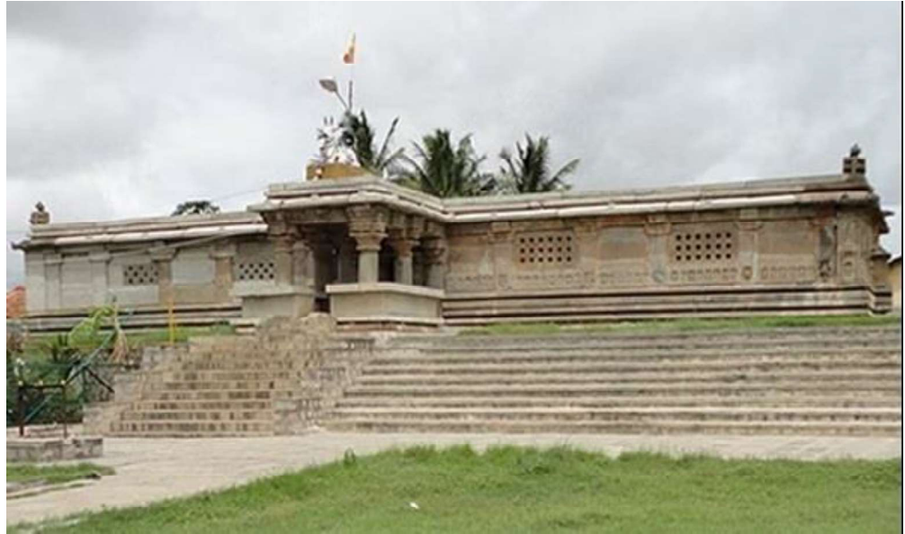
Picture No 4.22 – Sri Malleshwara Temple Aghalaya, K R Pet Taluk, Mandya District after conservation by SDMD Trust.
