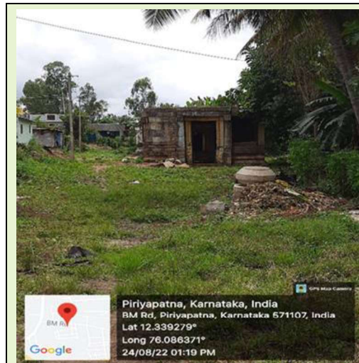
Picture No 4.11: No compound wall for Sri Channakeshava Temple, Periyapatna Taluk, Mysuru District.
