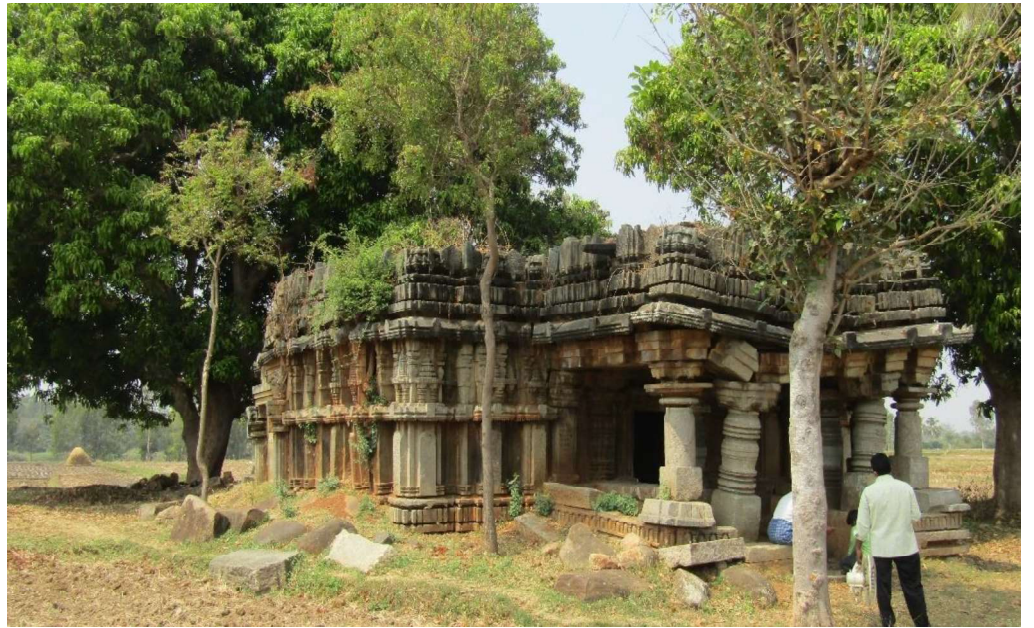
Picture No. 3.1: Dilapidated condition of an unprotected monument identified during survey at T Narsipura Taluk, Mysuru District.
