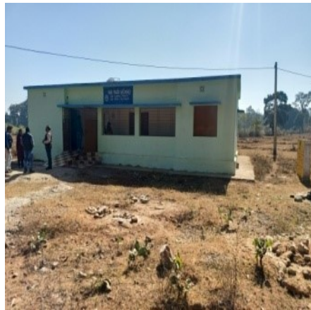
Picture 22: No approach road to the AWC at Mahulapada
