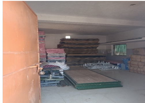
Picture-20: Renovated Laboratory, being used for storage purpose, at SDH, Udala
