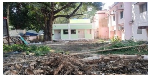
Picture-21: Toilet without approach road at SDH, Karanjia
