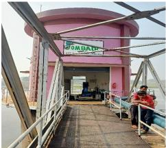
Picture-6: Floating jetty type intake well
