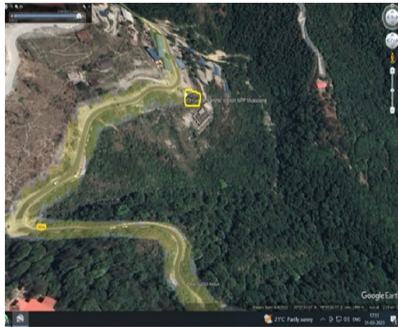
Photo-3.19: Aerial view of Secondary Storage facility NPP, near residential building Mussoorie (29 March 2023)
