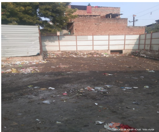
Photo-3.14: Secondary Storage facility in residential area at Shyam Nagar, Haridwar (02 February 2023)
