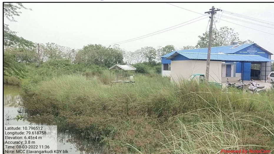
Exhibit 2.10: MCC established adjacent to water body in Elavangarkudi VP, Tiruvarur District
