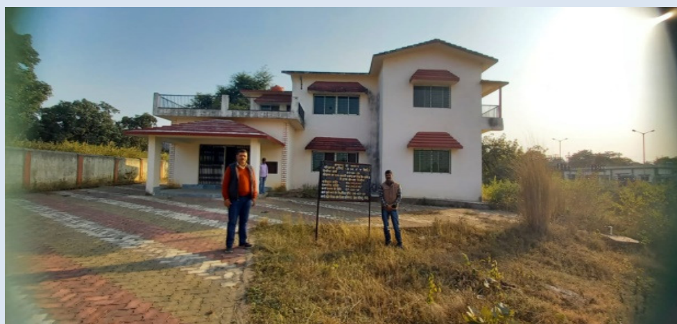
Picture 2: Dak-bungalow, McCluskieganj.
