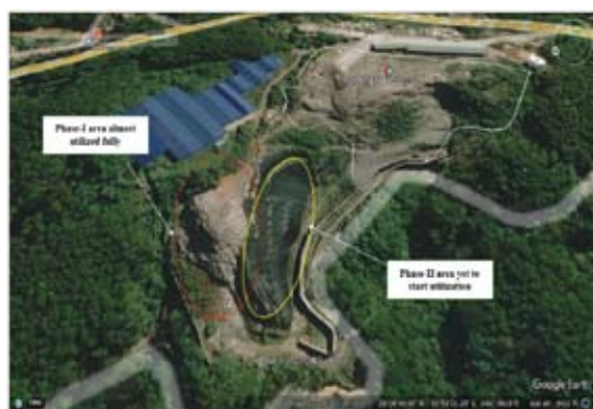
November 2020 image of Marten Landfill extracted from the Google Earth showing the Phase-I area almost utilized fully but Phase-II area was yet to be started utilization (black portion)
