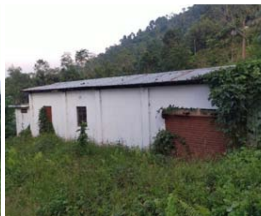
Exhibit 6.12: Unused office room
