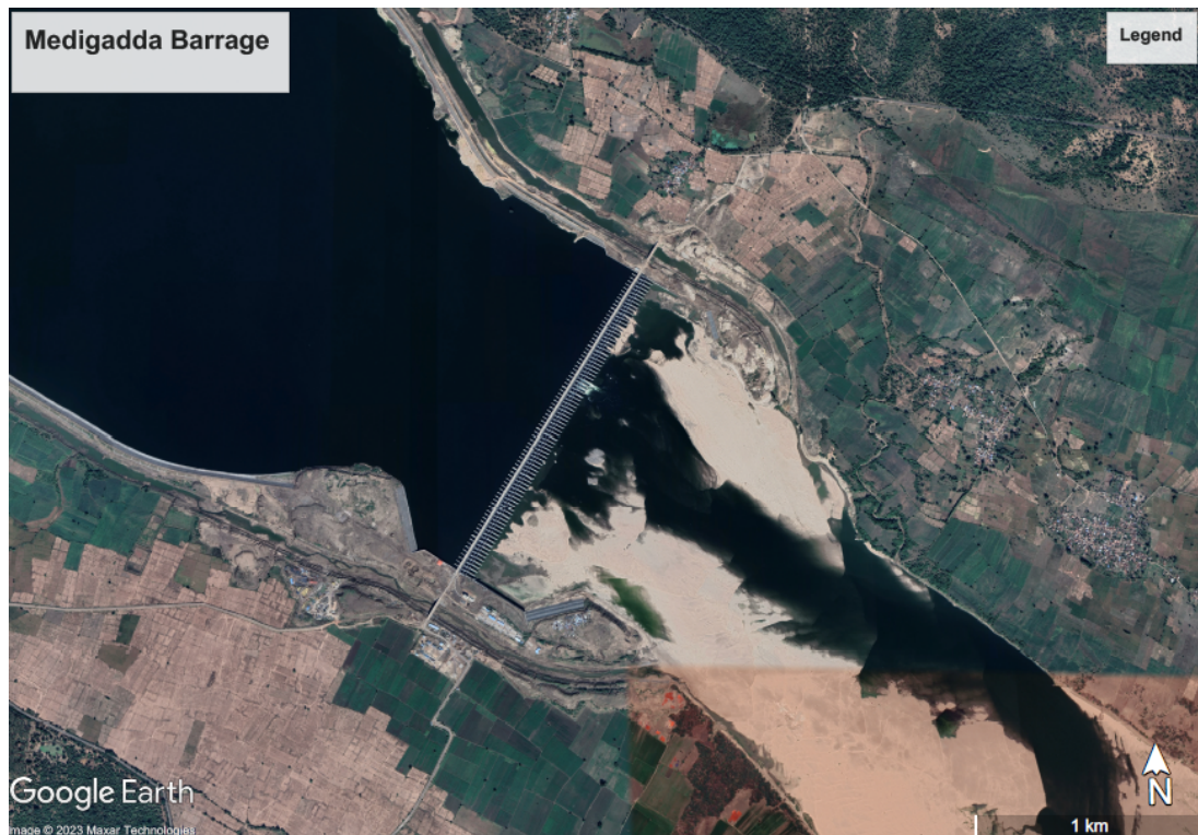
Figure 3.4 - Satellite image of Medigadda (Laxmi) Barrage
