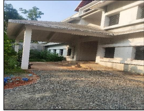
Figure 2.14: Academic block of SARBTM, Kozhikode – staircase not completed
