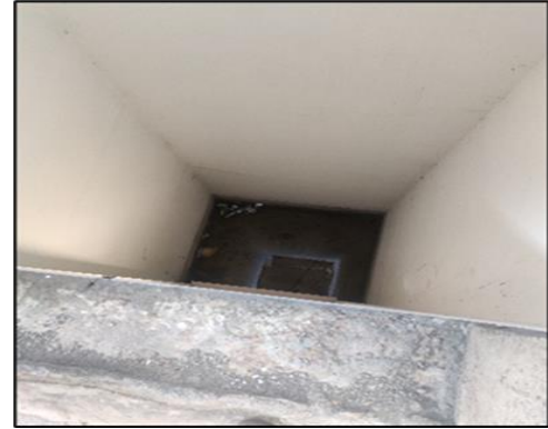
Figure 2.16: GHSS Parayanchery, Kozhikode - uncovered space for installation of lift
