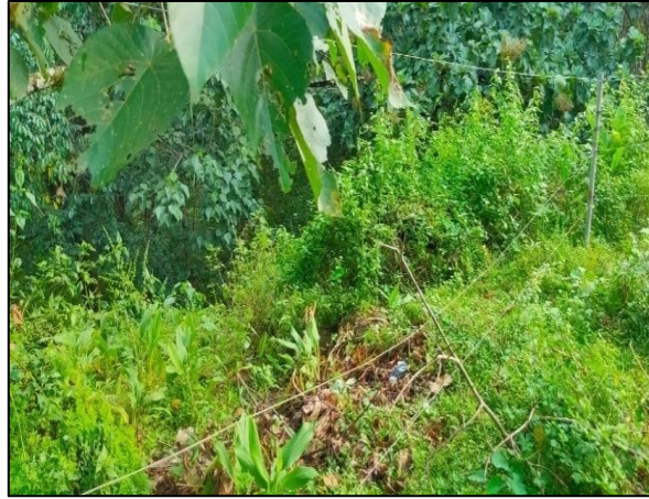
Figure 2.5: Non-maintained solar fence - Vadattupara in Malayattoor division (30 September 2021)
