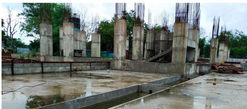
(Photo: Audit Team during Joint Physical Inspection, 26 July 2021)
