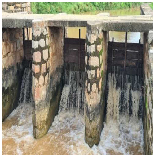
Water flow controlled by temporary gate (wooden planks) at the head of Islampur Branch of DCS
