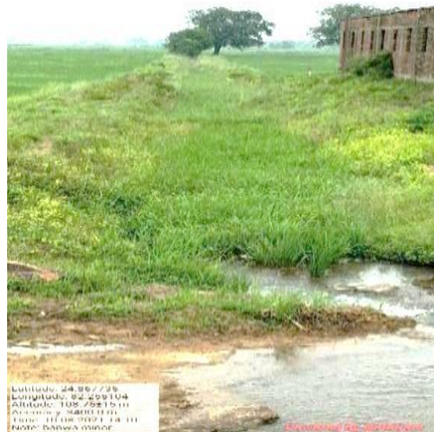
Silted Banwa minor of BCP (Last maintained; 2020-21)
