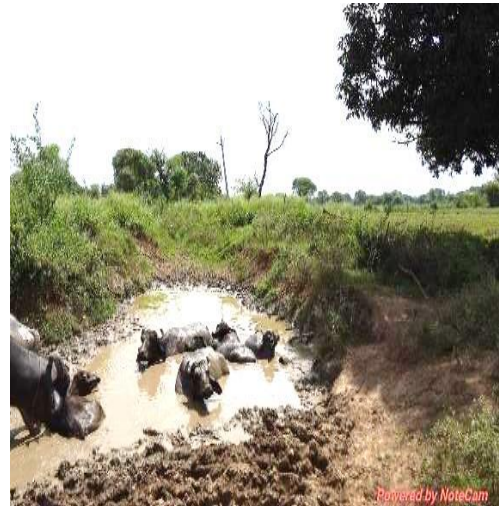
Silted Bilgaon minor in DCS (Last maintained; 2019-20)
