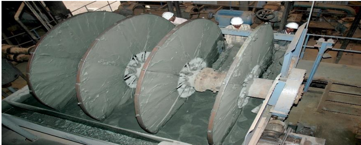
Figure 3.11 Operations in Concentrator Plant at Mosabani, Ghatsila
