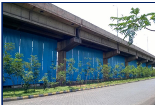
Picture 7.6 – Dust Barrier
