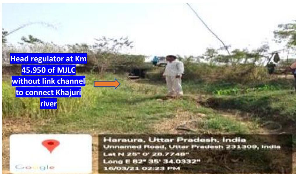
Without linking of head regulator to the river, diversion of water from MJLC to the river was not feasible. The farmers present during joint site visit also confirmed that no link channel was constructed.
