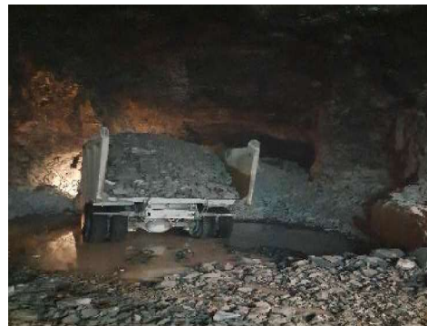
Excavation of Tunnel II using manual drill and blast method
