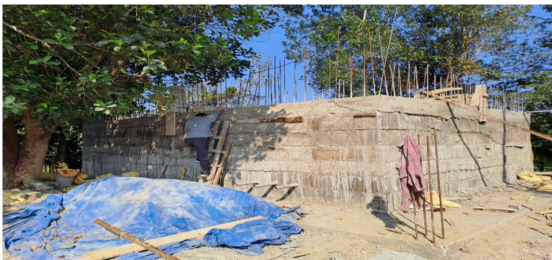
Picture: Construction of RCC reservoir 1,00,000 litres capacity at Buhchangphai
