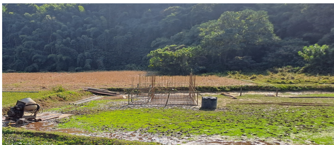
Picture: Construction of baffle wall sedimentation tank of water treatment plant at Buhchangphai
