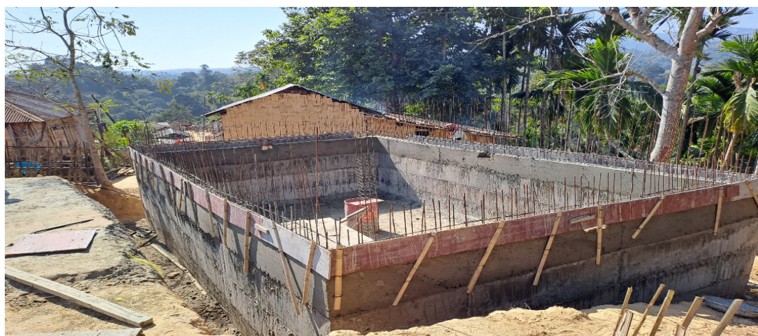
Picture: RCC reservoir of 1,00,000 litres capacity of the Saihapui 'K' Solar Pumping Water Supply Scheme at Saihapui
