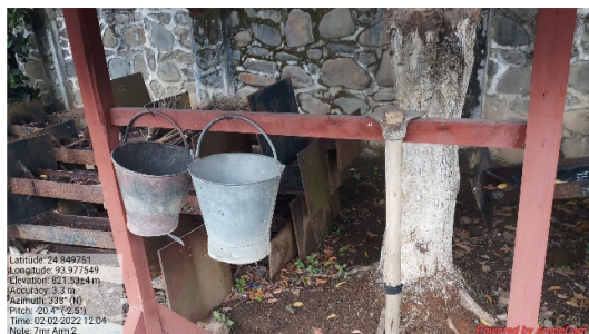
Installation of sand buckets without sand ( 7 th Battalion Manipur Rifles)
