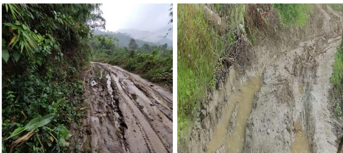
**Pic: Link-road without side drain and gravel**      **Pic: Link-road without side drain and gravel**
