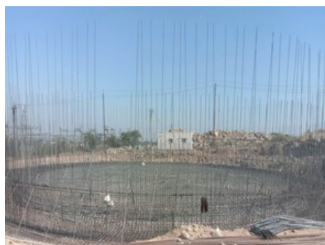
Incomplete compressed bio-gas plant at Jhiri, Ranchi.
