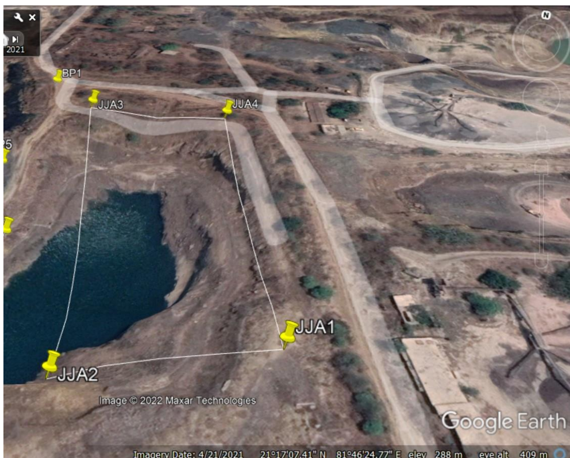
Figure-3.2 (a): Satellite image showing pit outside the approved co-ordinates ( khasra no. 1960, area- 0.971 hectare, village-Nardaha, Tahsil- Arang, District- Raipur, lease period- 25.09.2002 to 24.09.2032 ) Photo dated: April 2021, Source: Google Earth Pro
