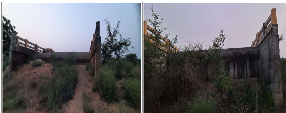
Physical status of both sides of new bridge (April 2022)
