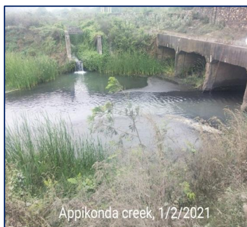
Discharge of untreated effluents into Appikonda Creek
