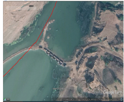
Photo dated: 03 January 2019 (Latitude- 25°04'35.20"N Longitude- 80°19'10.37"E)
