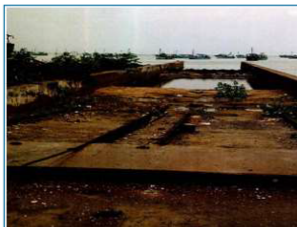
Exhibit 3.3: Slipway in Mallipatinam Fishing Harbour in Thanjavur
