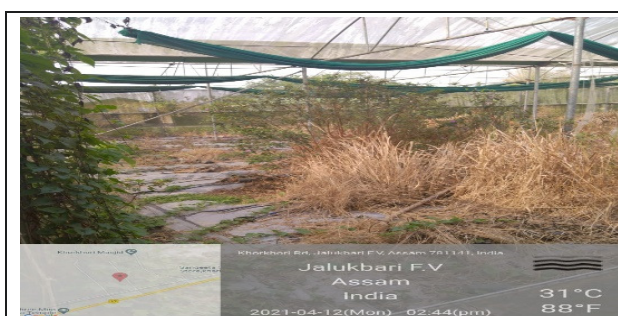
Green house (stated for root stock) roof damaged and full of bushes (12-04-2021)
