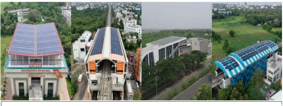
Figure 3.7: Roof top solar panels at Metro Bhawan and metro stations
