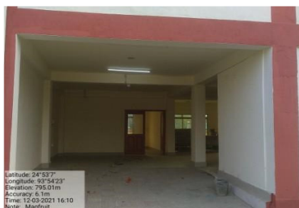
Collapsible shutter of unloading area not yet fitted
