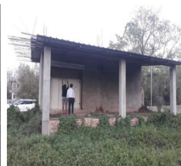
Idle Cold Storage unit at Kyamgei-Imphal East
