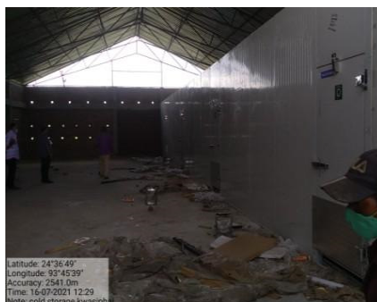
Incomplete cold storage unit at Kwasiphai
