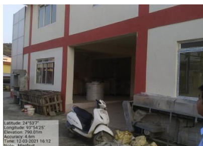
Collapsible shutter of loading area not yet fitted
