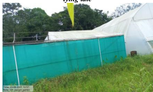
Badly damaged Low cost polyhouse at Panam Garden (Imphal East District) lying idle
