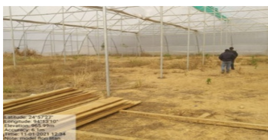
Polyhouse at Litan Centre (Ukhrul District) lying idle/unutilised
